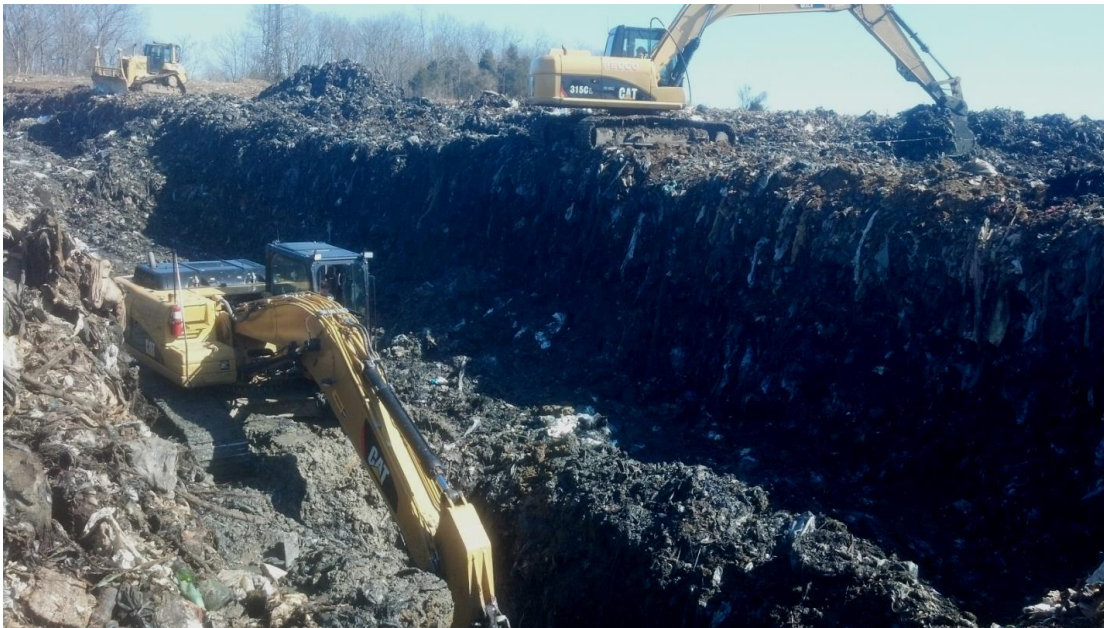
Contractors spent two days digging through trash and rock before uncovering the hidden spring 26 feet below the surface.
